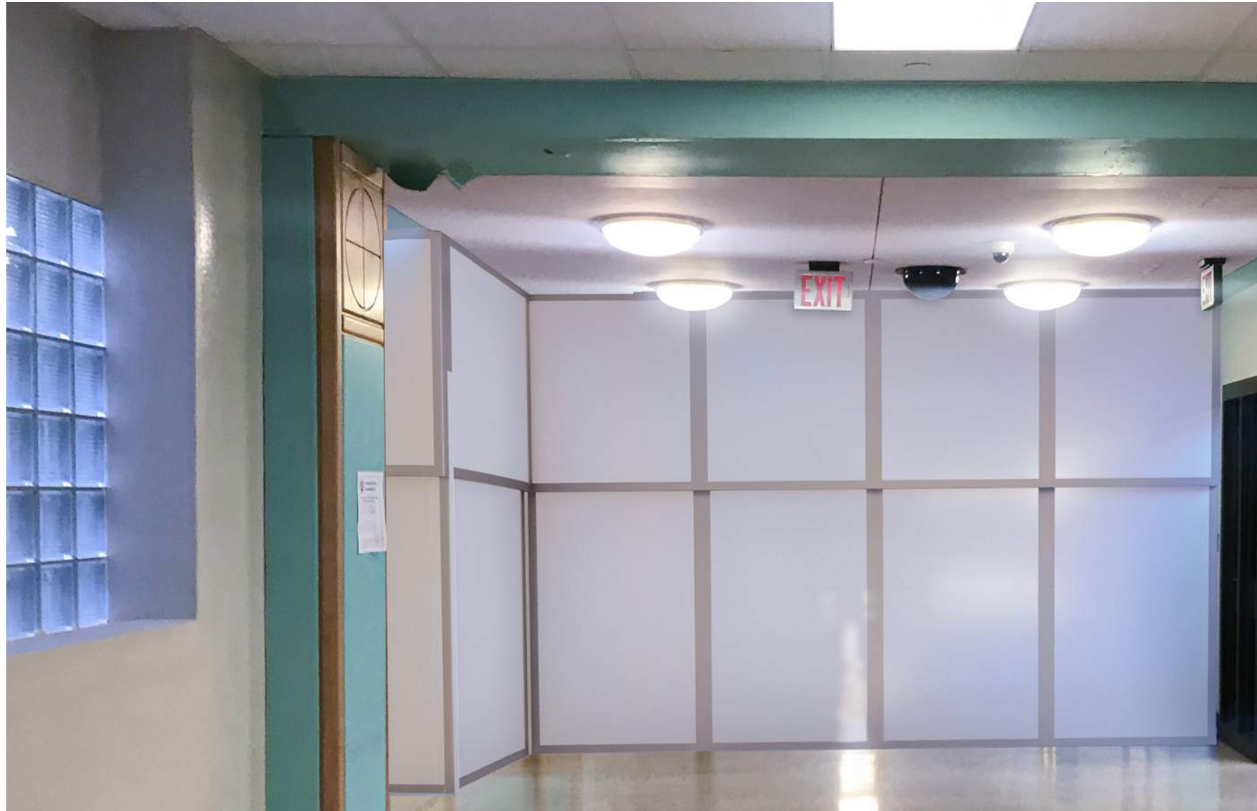
TEMPORARY PARTITION ACROSS HALLWAY EAST BUILDING
